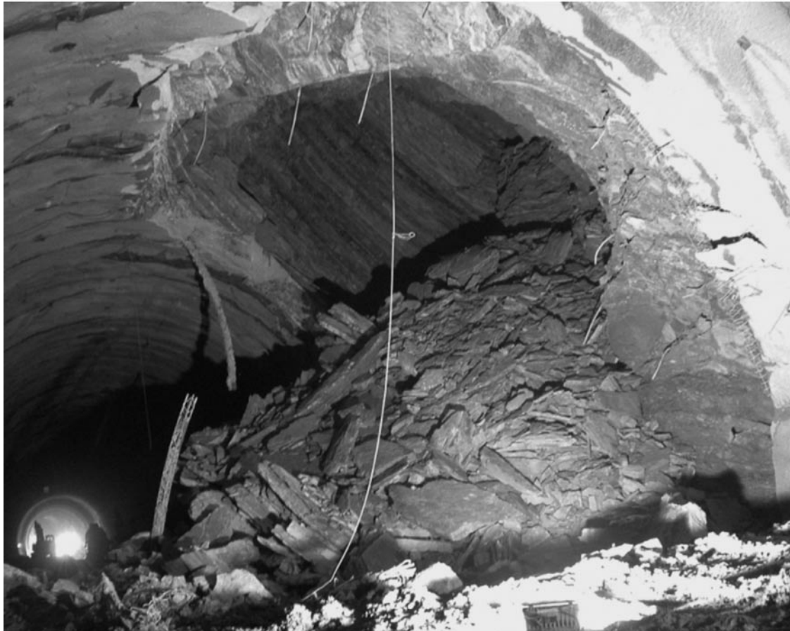
Fig. 8 Failure of Tunnel Section Induced by Unstable Key Block
